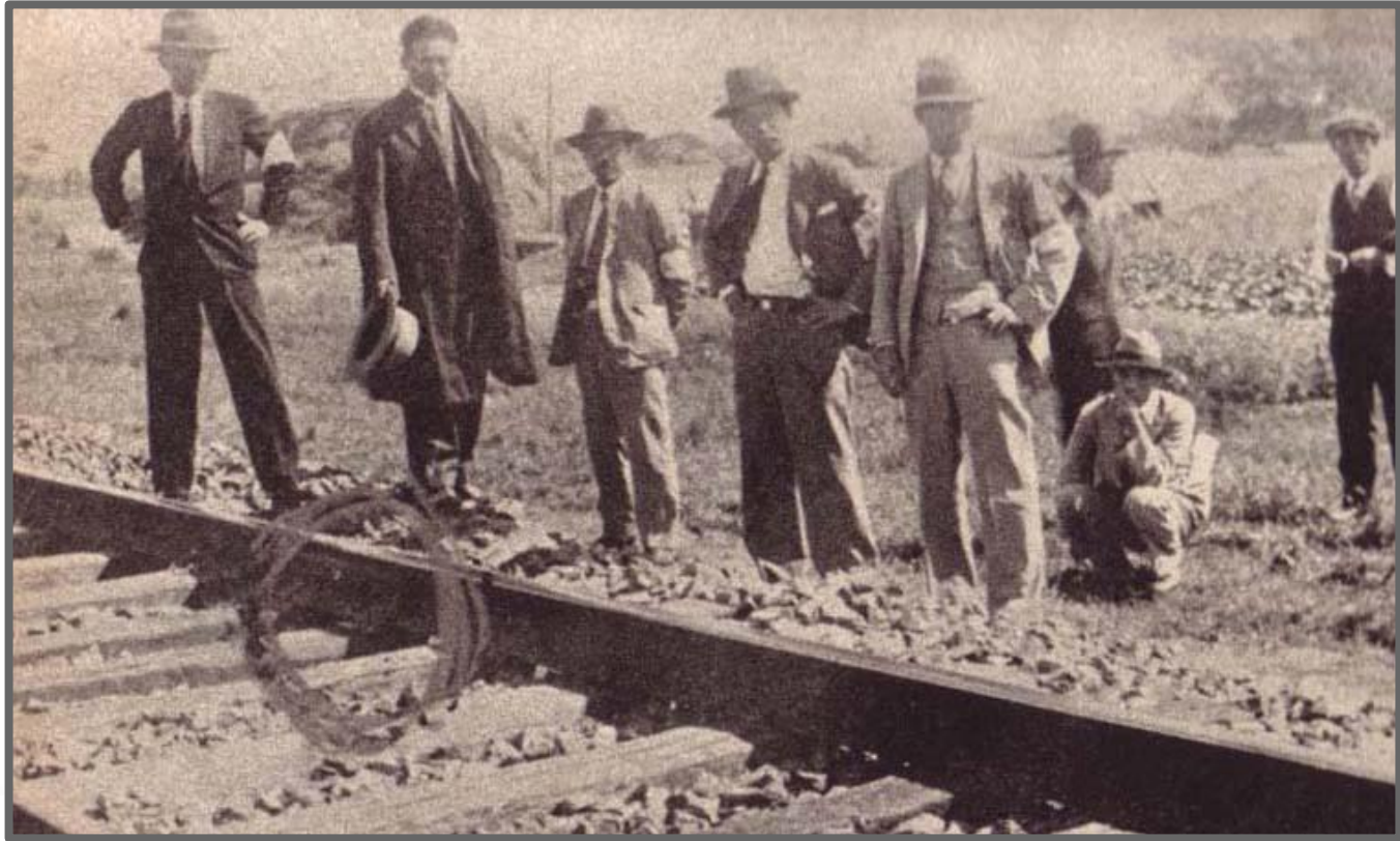
Inspecting the Railroad - little damage done.
